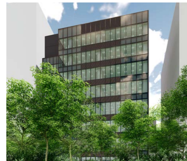
北側外観 Exterior view of the north side
